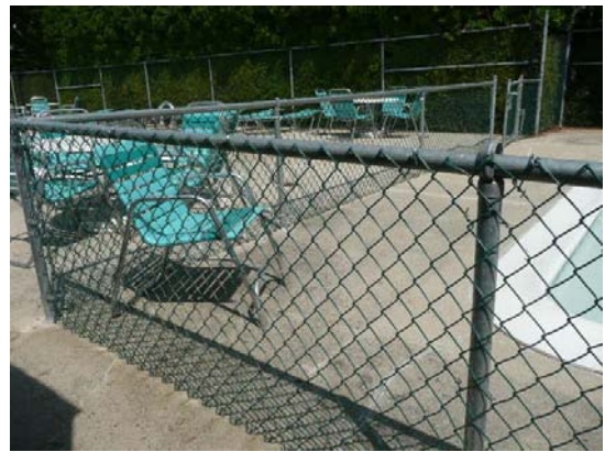
3' chain link fence, vinyl coated
