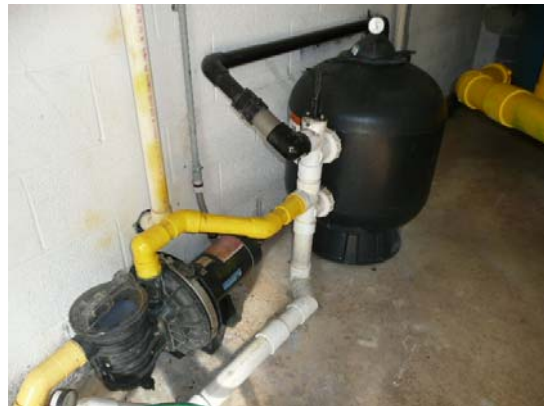
Baby pool filter and pump
