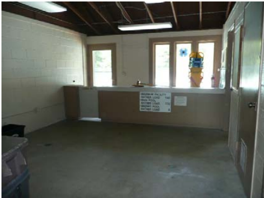
Open area with millwork for guards
