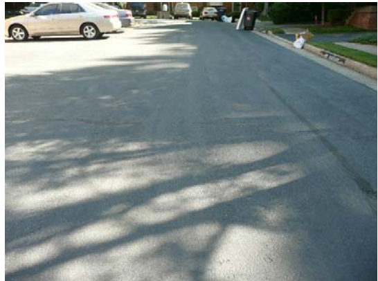
Ashley Glen Road asphalt
