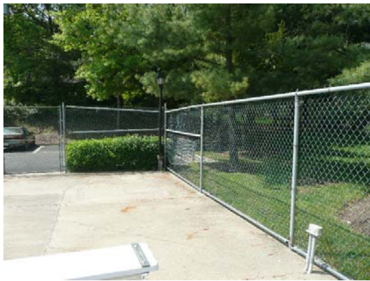
6' chain link fence, vinyl coated
