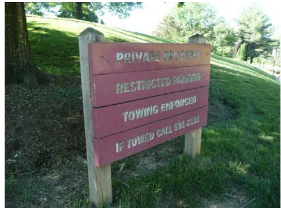
Wood signage; typical condition
