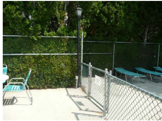
Light pole; typical
