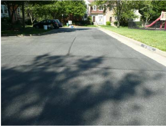
Trammell Court asphalt
