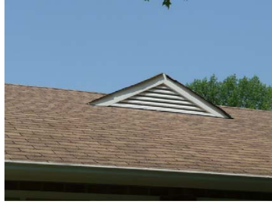
Pool building roof
