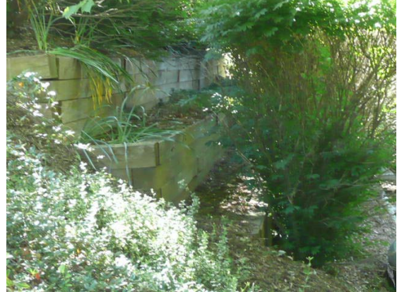
Wood retaining wall, Hancock Forest Terrace
