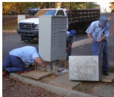
A new mailbox being installed
