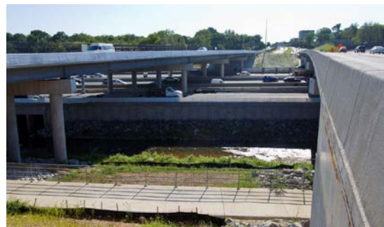
New Little River Turnpike Bridge, looking east
