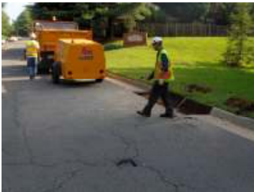
Crews fix curbs and cracked pavement in our neighborhood.
